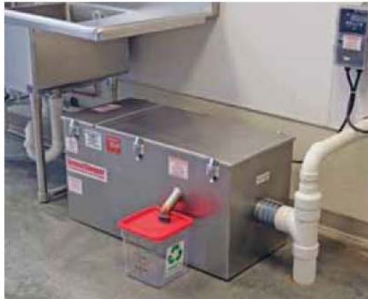
Figure 2.13b: Grease Interceptor–Installed
